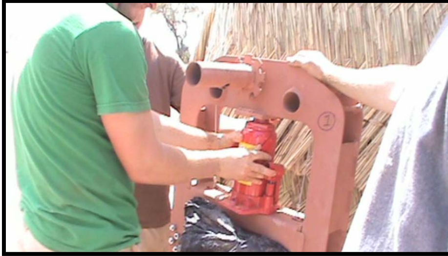
Positioning the 20-Ton Hydraulic Jack into its Groove in the Center of the Press
