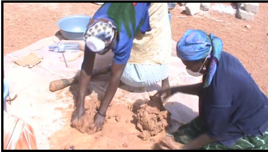
Wet-Mixing the Clay, Rice Husk and Water Mixture
