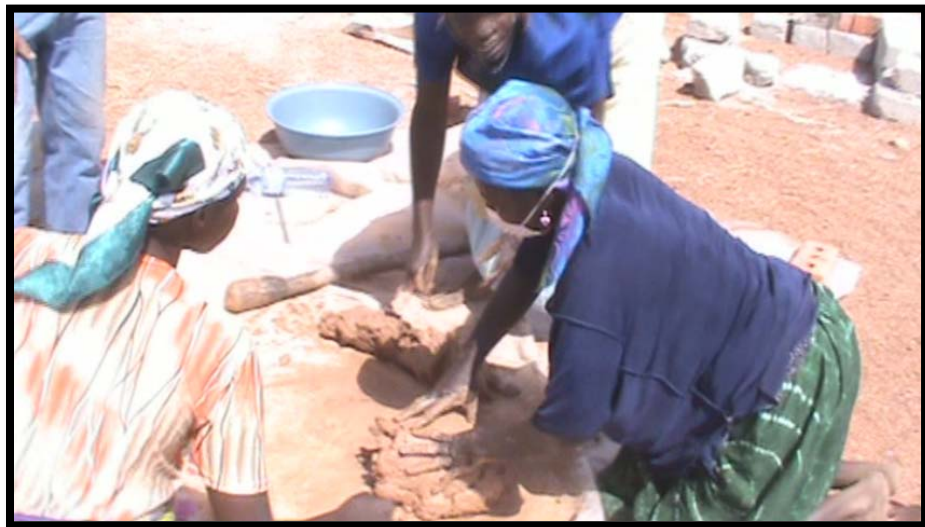
Wedging the Wet Clay, Rice Husk and Water Mixture
